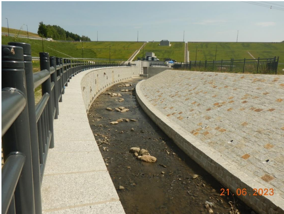
Phot. 17. Restoration of the bottom structure of the new bed of the Nysa Kłodzka River by placing large stones in the bed (item no. 58 of EMP).
