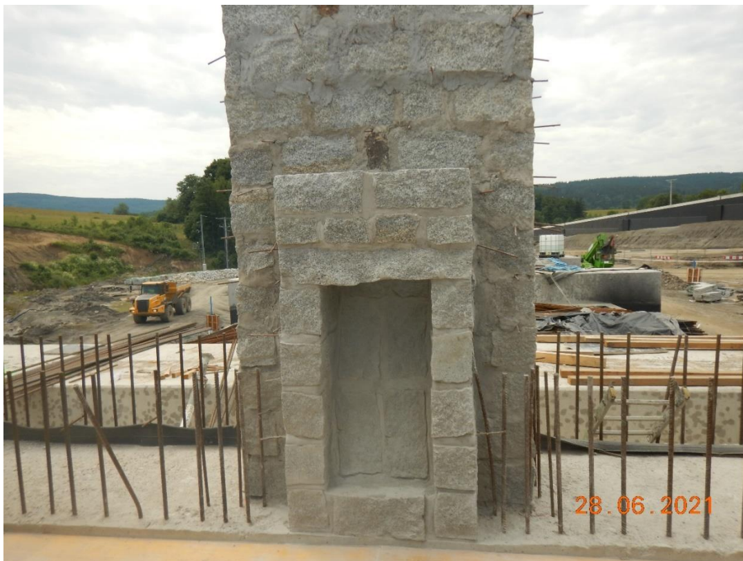
Phot. 11. Installation of chambers for bats in chimneys of the tunnel of the reservoir's dam.
