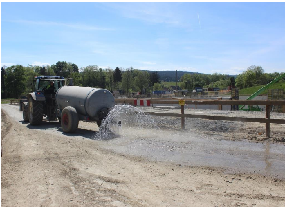
Phot. 6. Spraying dusty road surfaces (item no. 89 of EMP).
