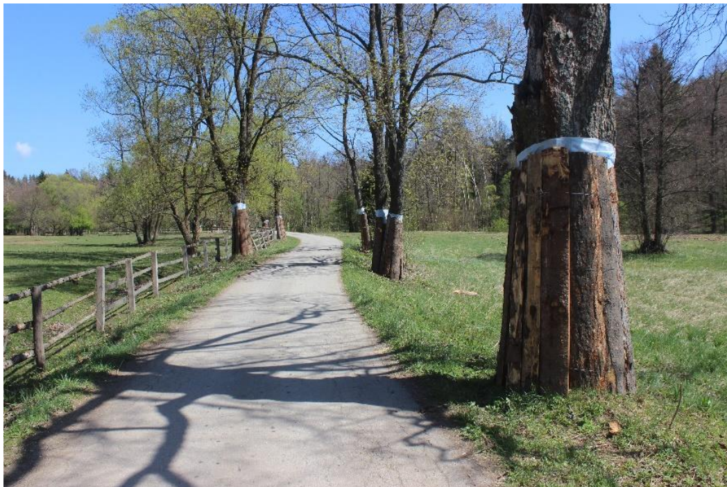
Phot. 12. Secured trunks of the trees not intended for felling at the Construction Site (item no. 20 of EMP)
