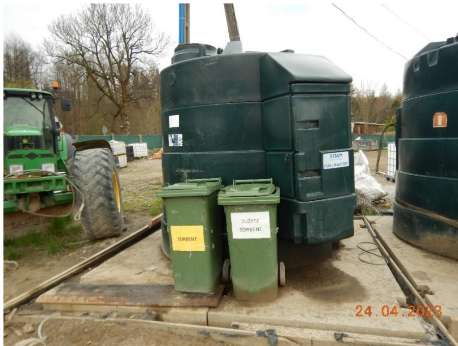
Phot. 5. Vehicle refuelling point at the construction site facilities - protected from the ground and equipped with sorbent (item no. 80 of EMP).
