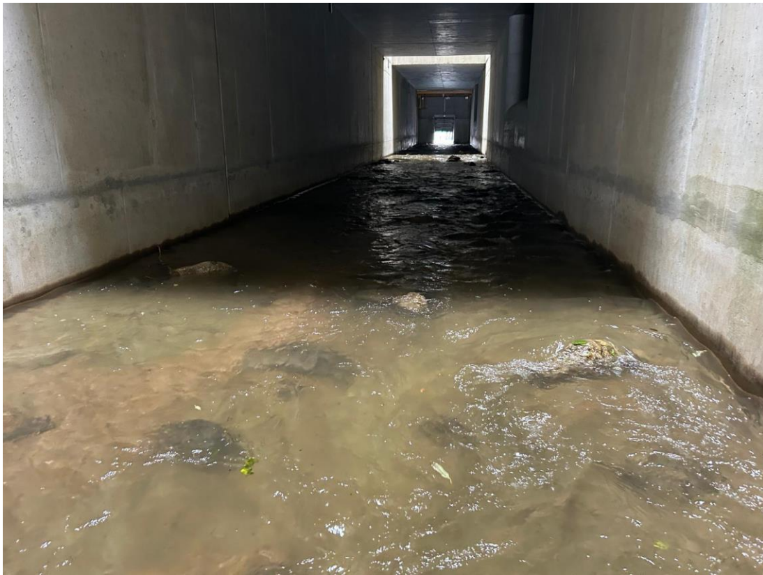
Phot. 19. Tunnel under the reservoir dam – stones deposited in the bottom visible (item no. 58 of EMP).
